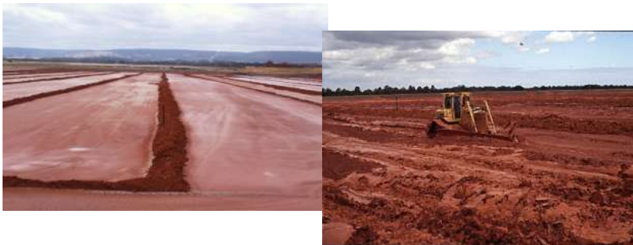
Figure 3 Spreading the slurry, and ploughing using a D6 Swamp Dozer to enhance the drying rate
